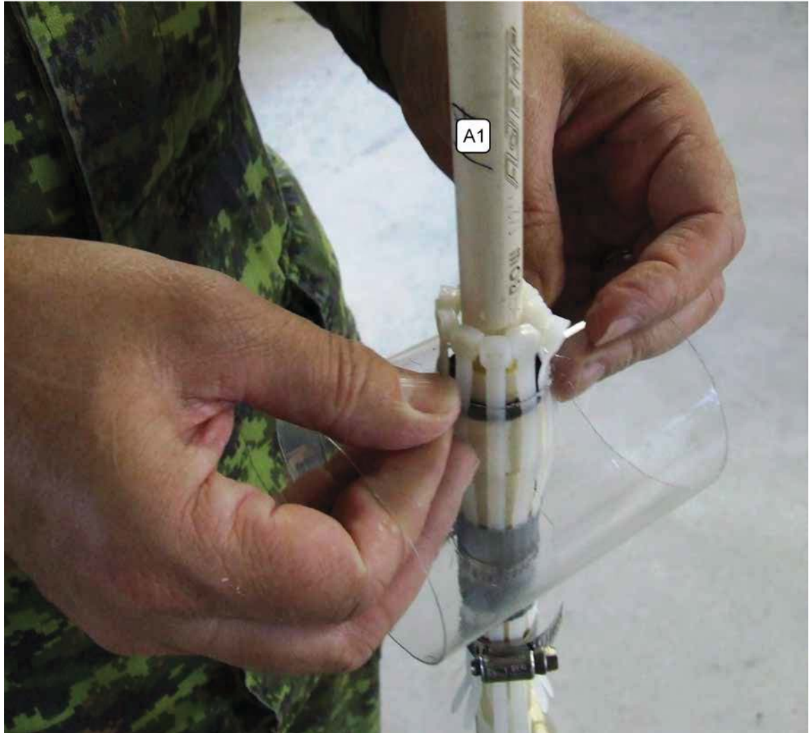
Figure 28-A Sliding the Spring over the Cable Ties
